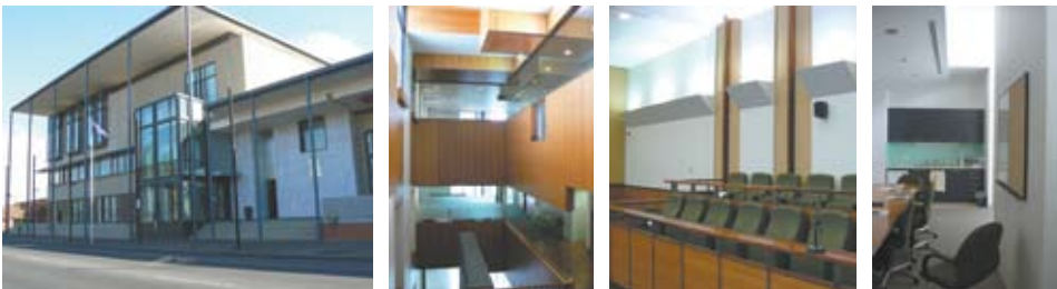
Photos (left to right): (1) Ballarat Court Complex entrance; (2) The internal staircase; (3) The jury box; (4) Jury deliberation room.
