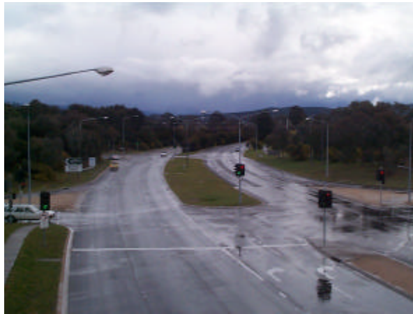
Figure 3 Hindmarsh Drive, between the suburbs of Waramanga and Weston.
